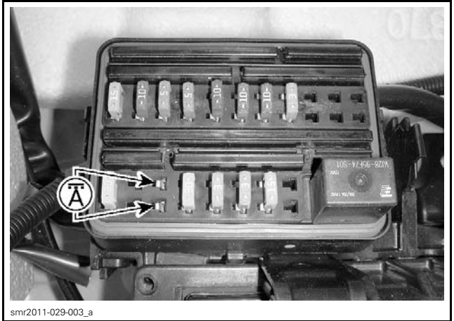
CHARGING SYSTEM FUSE REMOVED
