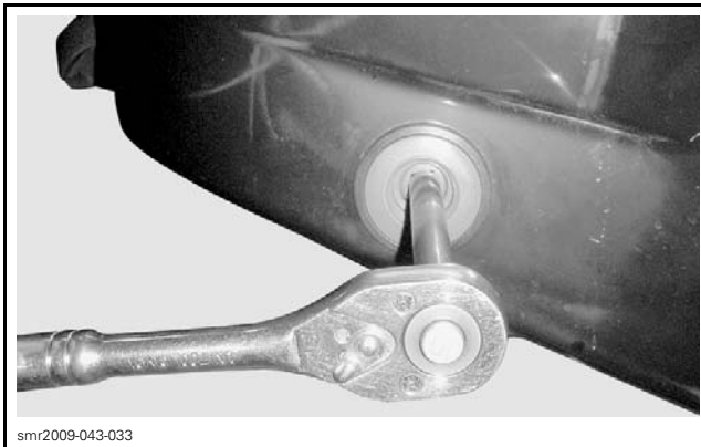
DRAIN NECK REMOVAL
